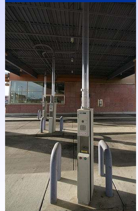
Pneumatic Tube at the Drive Through Bank
